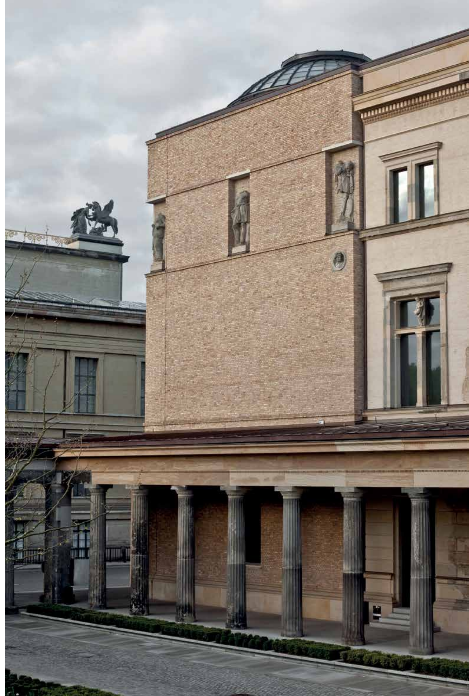
Fachada sur-este. © Ute Zscharnt for David Chipperfield Architects
