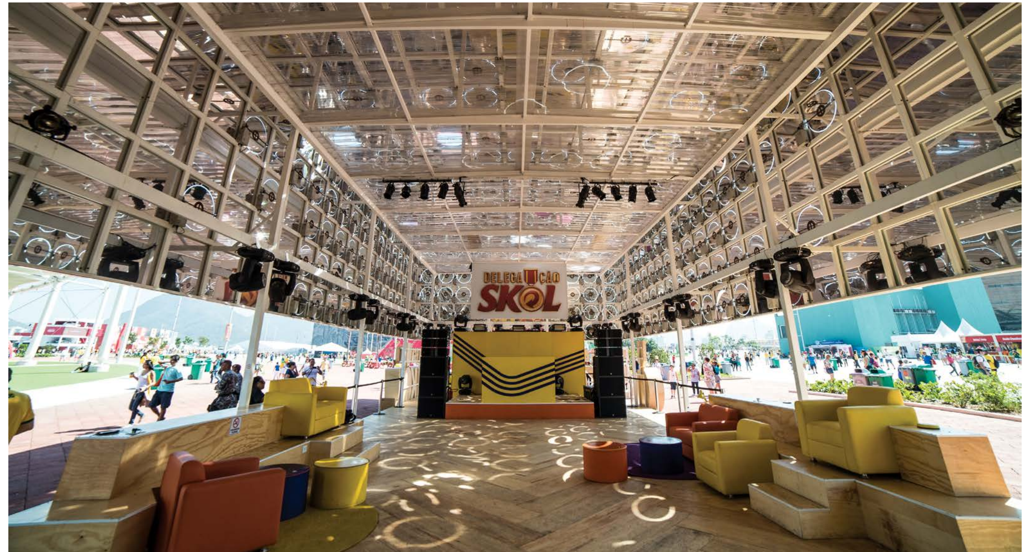
Vista interior del pabellón / Interior view of the pavilion. © Fernanda Ligabue & Rafael Frazão
